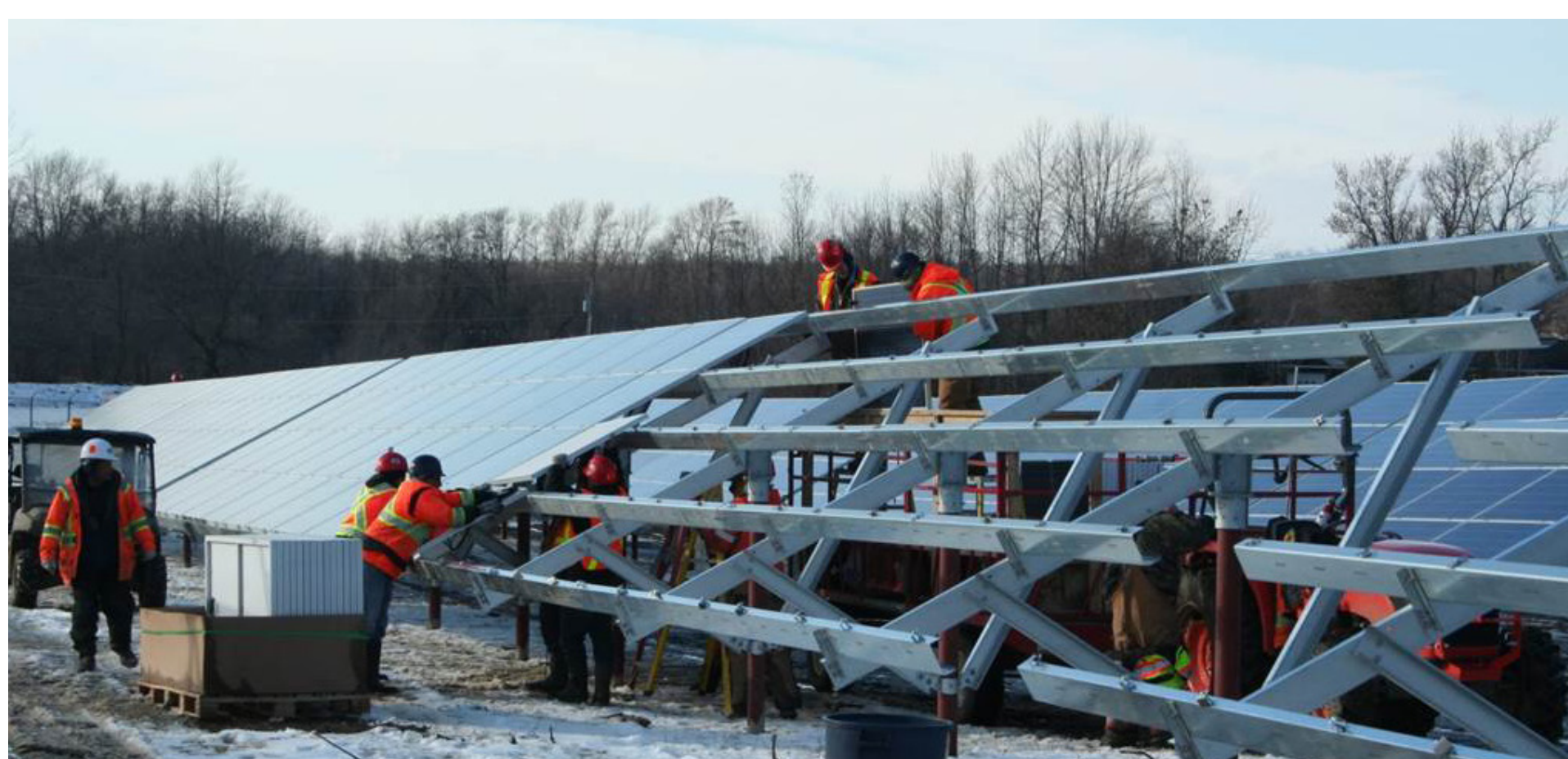
Module Installation
