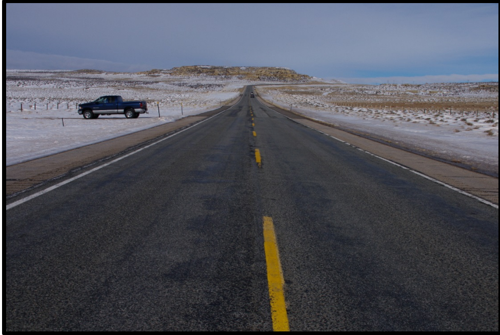
Figure 48. Photograph WY 487/Access 4 Looking North
