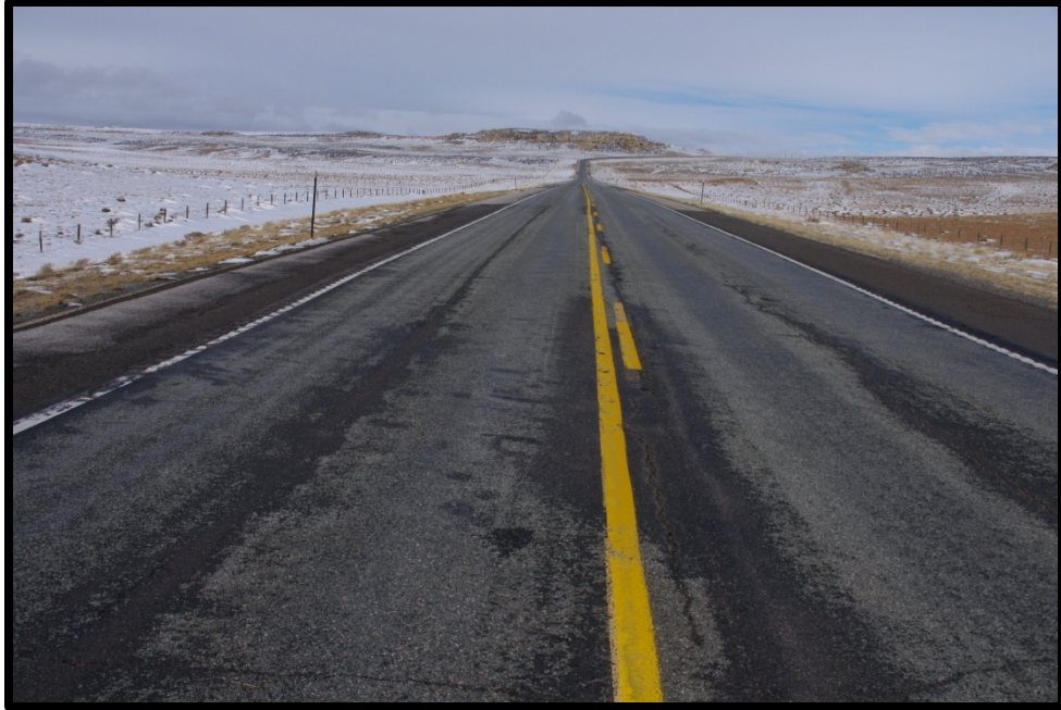
Figure 45. Photograph WY 487/Access 3 Looking North
