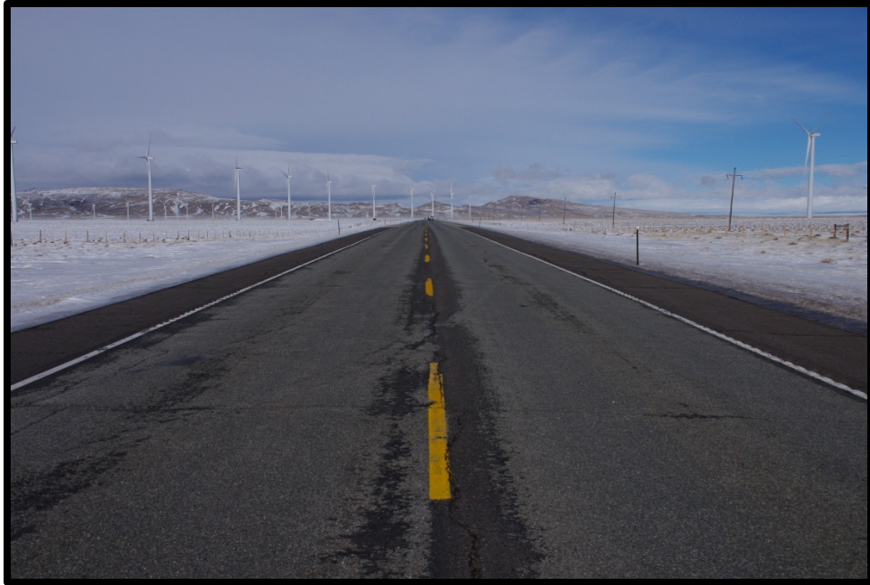
Figure 34. Photograph WY 487/CR 294 Looking North
