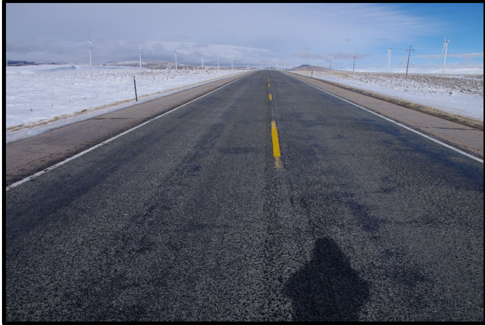
Figure 54. Photograph WY 487/Access 6 Looking North
