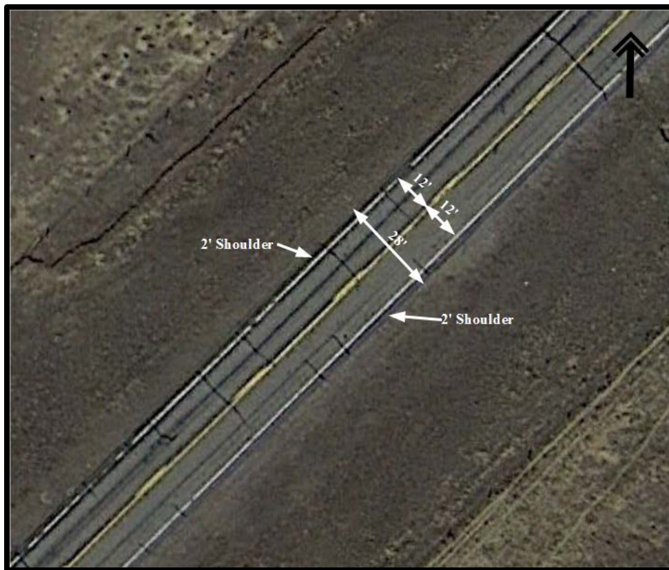
Figure 8. Aerial View WY 13
