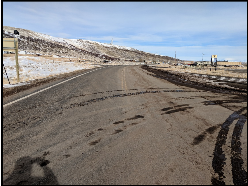
Figure 17. Photograph Westbound I-80 Ramp with WY 13 Looking North
