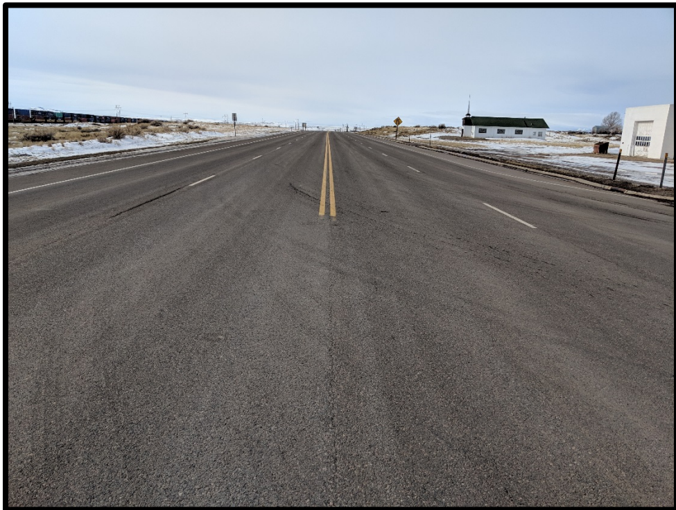
Figure 29. Photograph US 30/WY 487 Looking West
