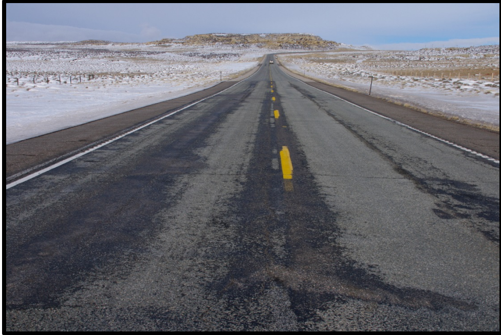
Figure 51. Photograph WY 487/Access 5 looking North
