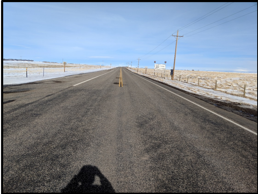
Figure 22. Photograph US 30/WY 13 Looking Northbound
