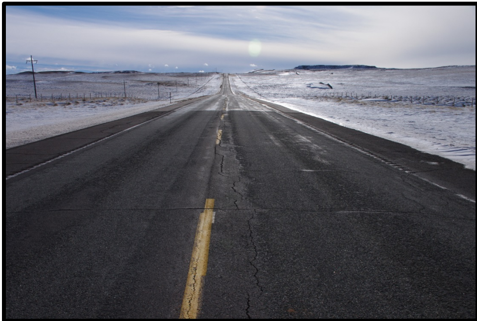
Figure 35. Photograph WY 487/CR 294 Looking South
