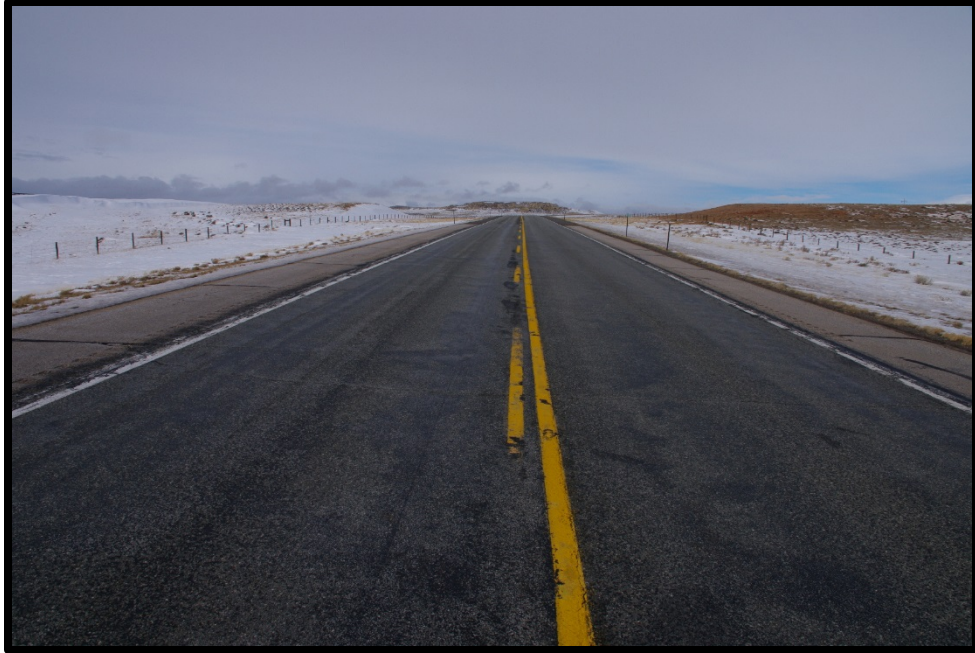
Figure 42. Photograph WY 487/Access 2 Looking North
