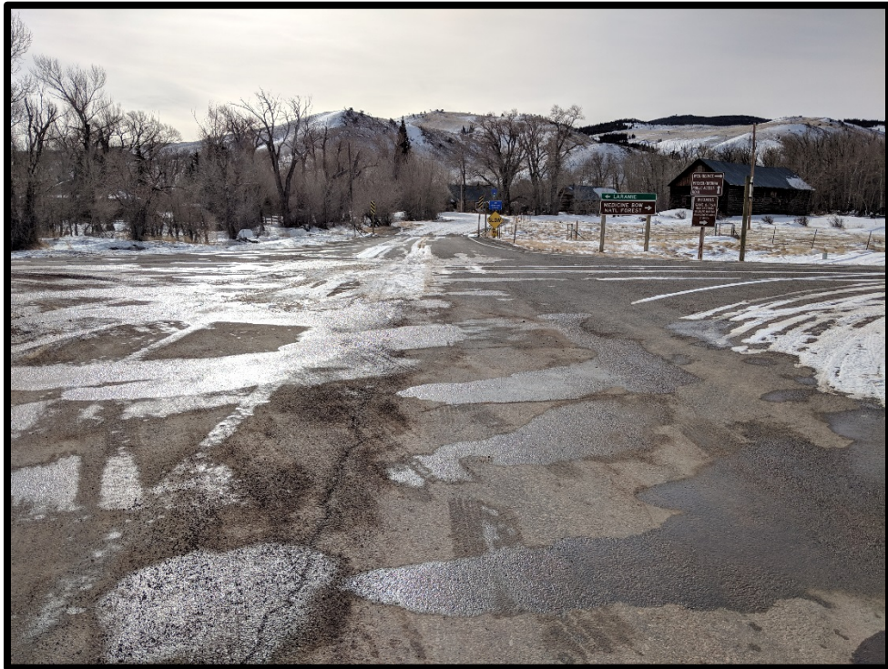
Figure 20. Photograph Eastbound I-80 Ramps with WY 13 Looking South
