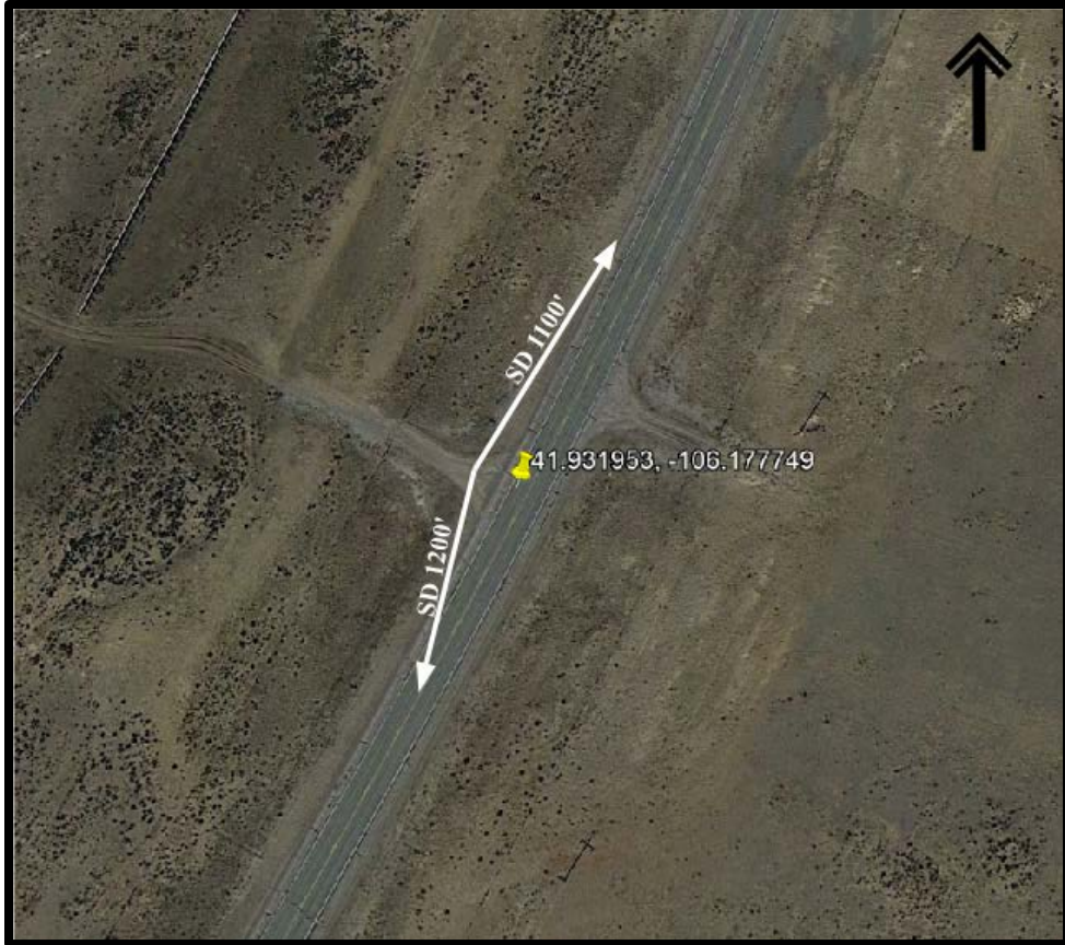
Figure 38. Aerial View Access 1
