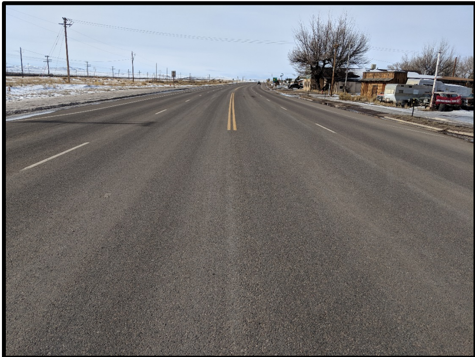
Figure 26. Photograph US 30/CR 1 Looking West
