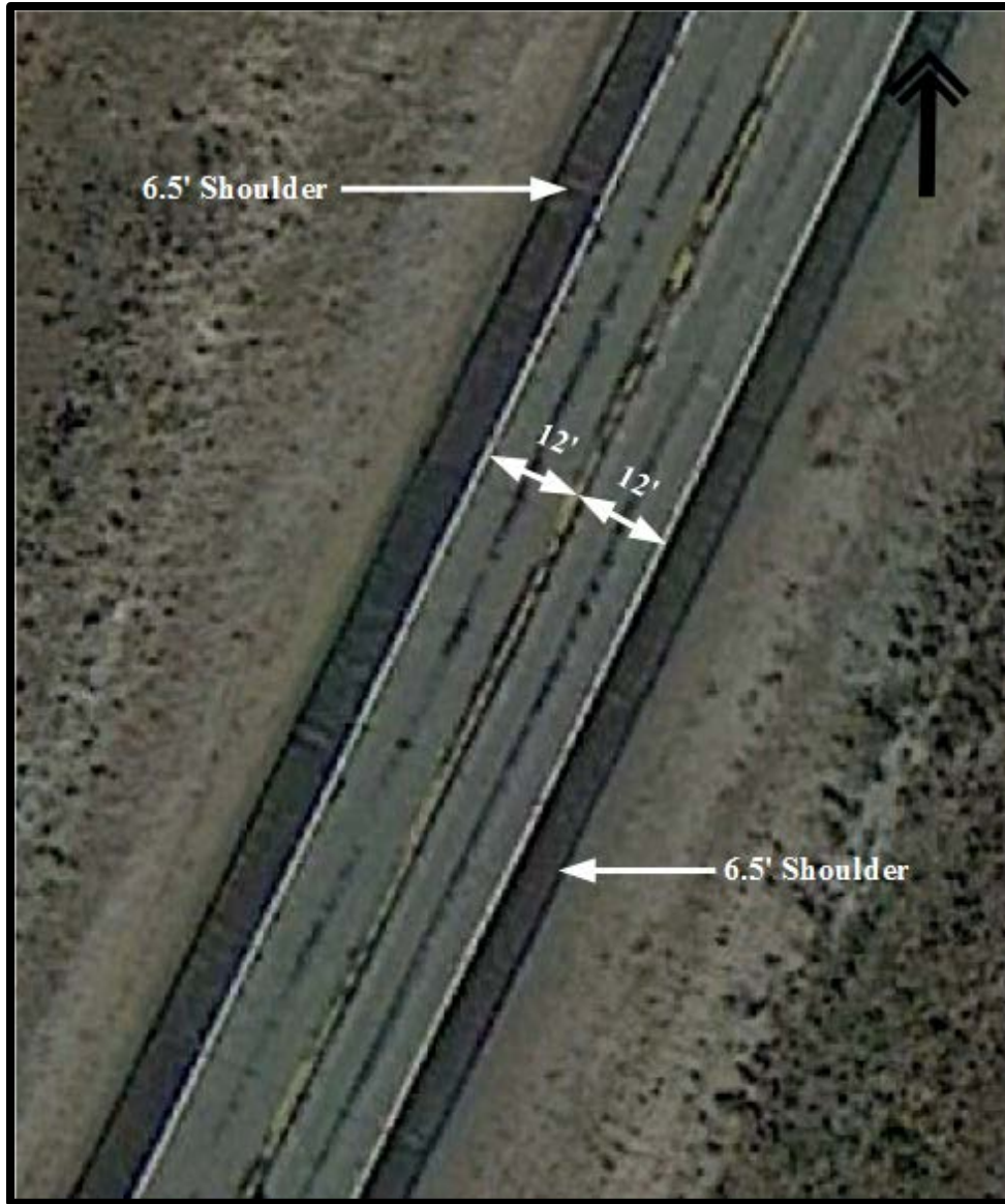
Figure 11. Aerial View WY 487
