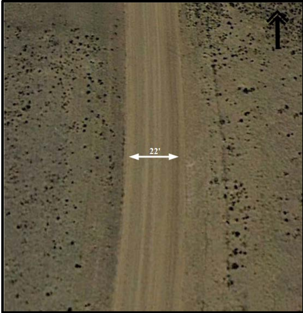
Figure 13. Aerial View CR 1 South of CR 3
