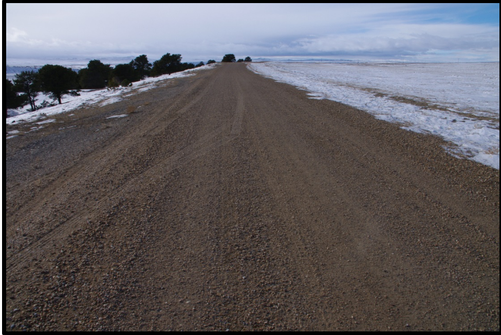
Figure 60. Photograph CR 262/Access 8 Looking West
