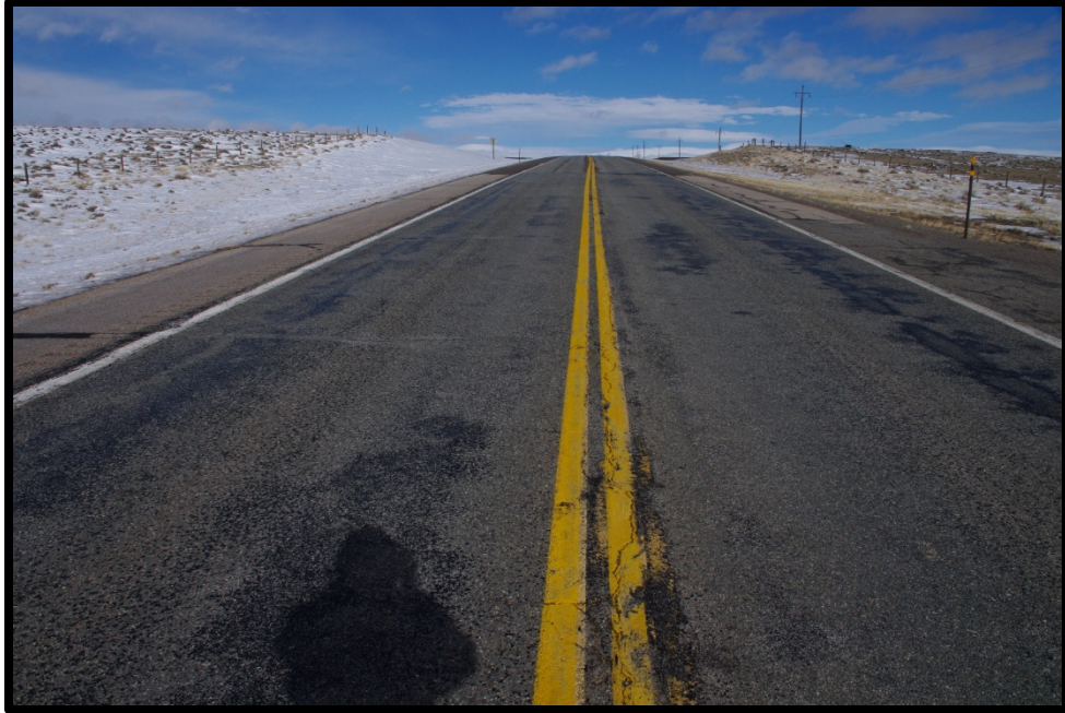
Figure 31. Photograph WY 487/CR 262 Looking North
