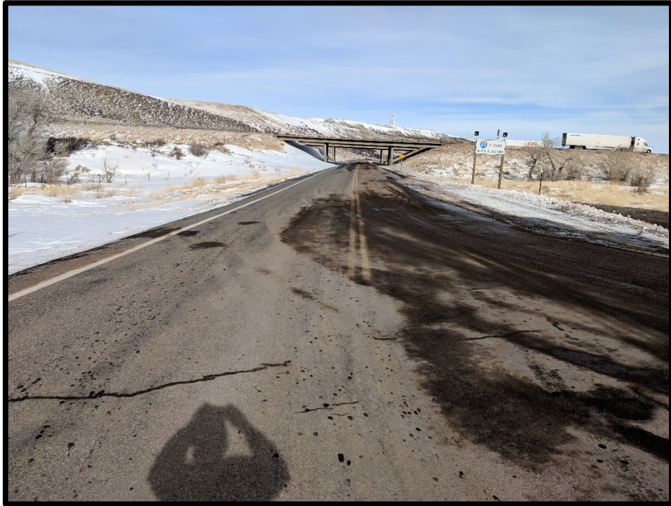
Figure 19. Photograph Eastbound I-80 Ramp with WY 13 Looking North
