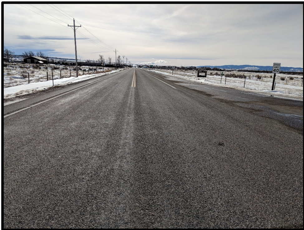
Figure 23. Photograph US 30/WY 13 Looking Southbound
