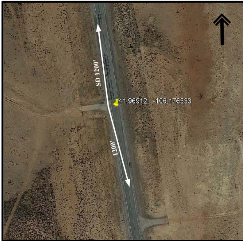
Figure 50. Aerial View Access 5
