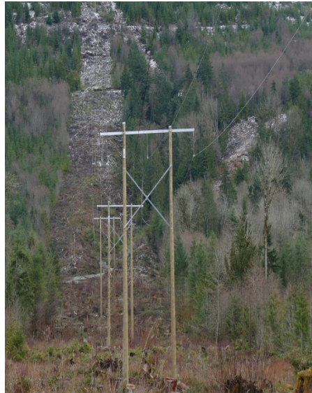
Figure 3. Picture of Typical H-frame Transmission Structure
