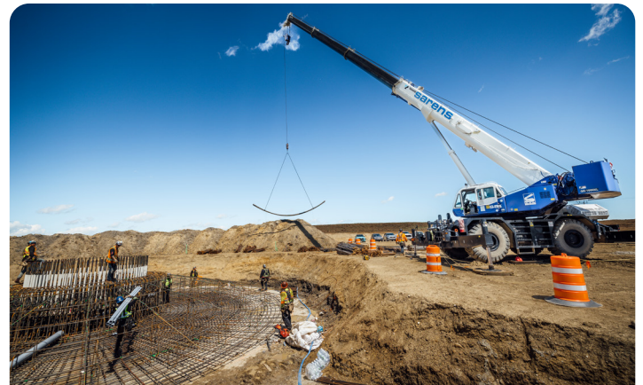
Bolt cage assembly for a turbine foundation.
