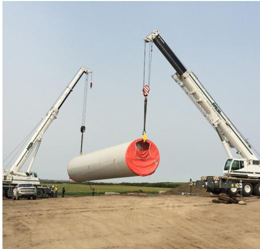
**Turbine Assembly.** Turbines are assembled and installed using cranes.
