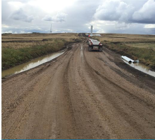
**Civil Works.** The ground area is prepared and construction of roads and laydown areas begin.
