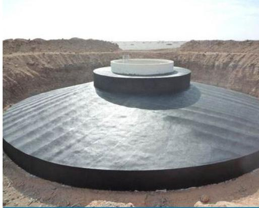
**Turbine Foundations.** Foundations for the wind turbines are constructed from concrete and steel.
