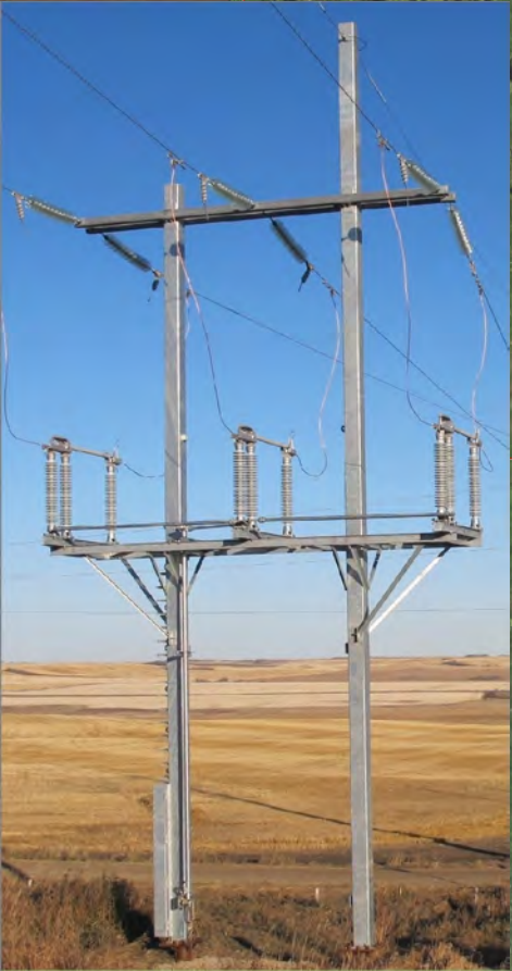
Example of 144 kV switch structure
