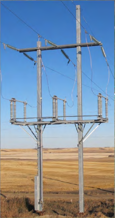
Example of 144 kV switch structure
