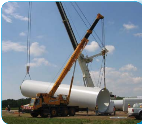
Wind Turbine Installation
