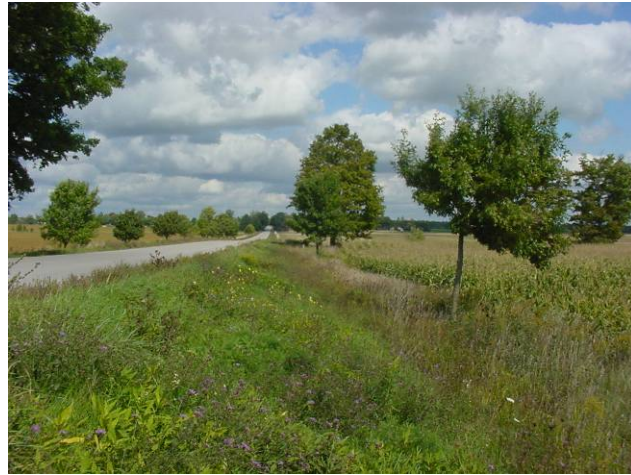
Plate 50: view to northeast, fill slope disturbance along paved and improved McNabb Line.
