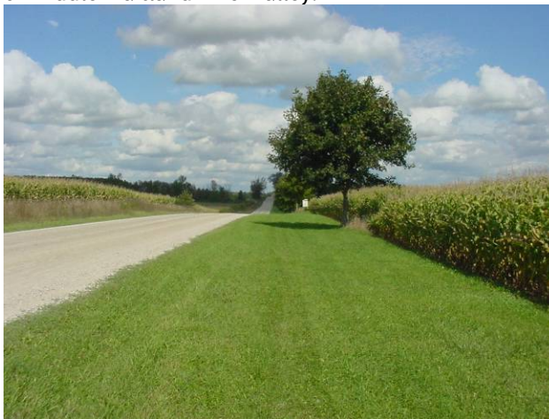
Plate 65: view to northeast, wide, gentle fill slope disturbance along gravelled McNabb.
