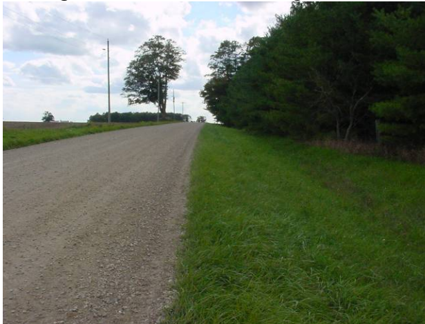
Plate 99: view to southeast, ditch and fill slope disturbance along Johnston Line. Historic farmstead at right.
