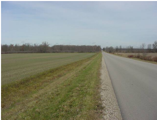
Plate 43: view to northeast, fill slope and ditch disturbance along paved and improved McNabb Line.
