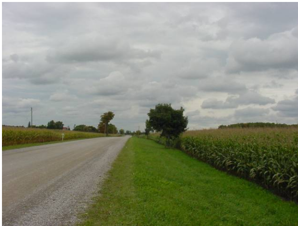
Plate 9: view to northeast, fill slope disturbance along Manley Line. Level terrain near farmstead.
