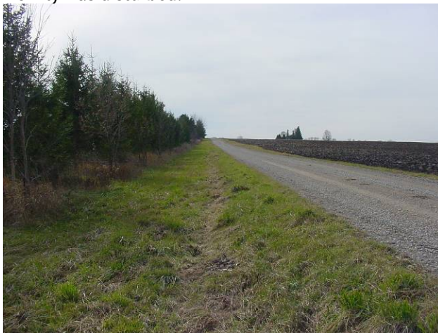
Plate 35: view to southwest, disturbed fill slope along Manley Line.
