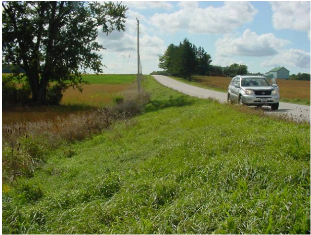
Plate 49: view to southwest, fill slope on low ground near drainage ditch at intersection with St. Michaels Road.
