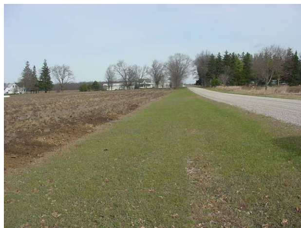
Plate 24: view to northeast, fill slope disturbance along Manley Line.
