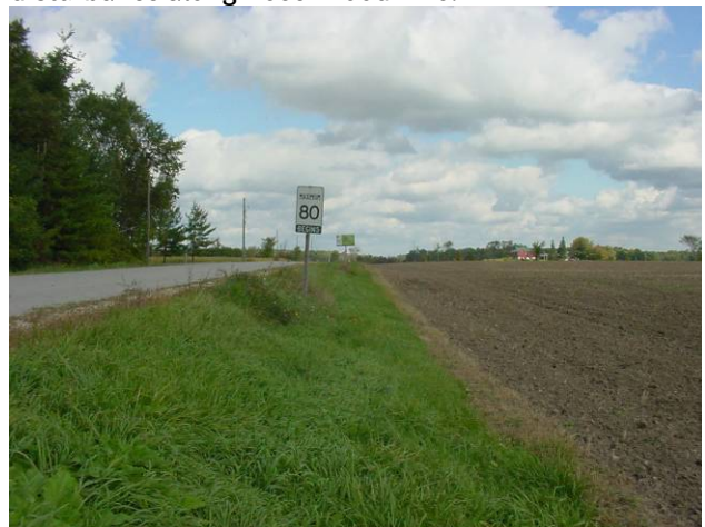
Plate 42: View northeast, steep fill slope along paved and improved McNabb Line.
