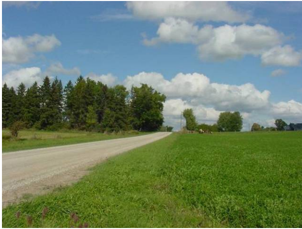
Plate 73: view to northeast, fill slope and ditch disturbance along southeast side of McNabb.
