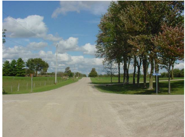
Plate 76: view to northeast, ditch and fill slope disturbance along McNabb, north of Cardiff Road intersection.
