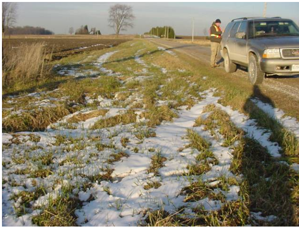
Plate 31: view to northeast, wide, gentle fill slope along Manley Line.
