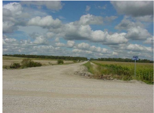
Plate 94: view to northeast, ditch & fill slope disturbance along Johnston Line through low and level terrain.
