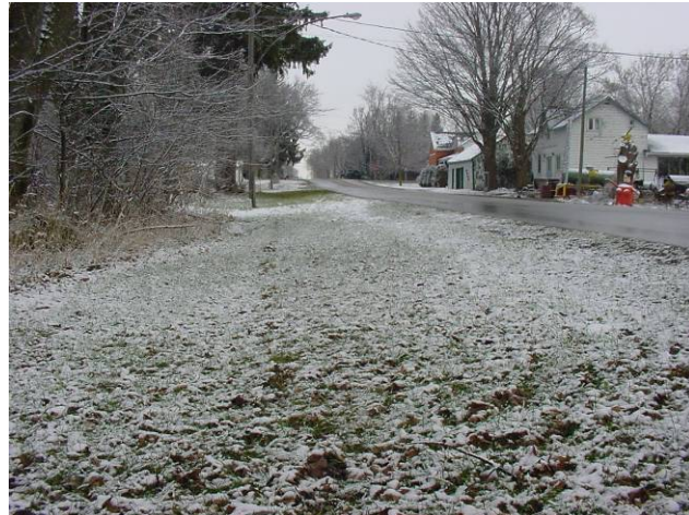
Plate 52: view to northeast, from south limit of hamlet of Cranbrook, along northwest side of McNabb. Fill slope disturbance in study corridor.
