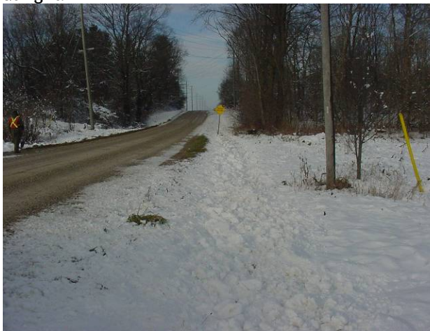
Plate 101: view to northwest, ditch, fill slope and cut slope disturbance along Centre line Rd.
