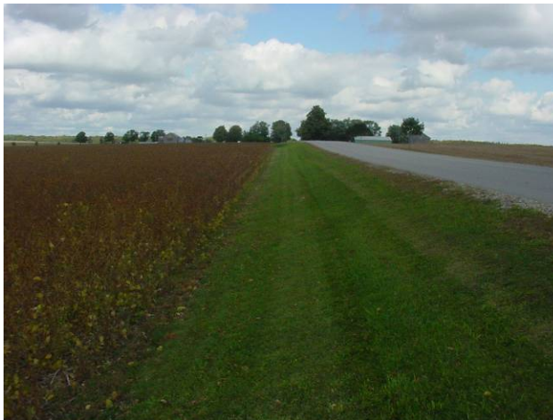
Plate 45: view to northeast, fill slope disturbance along paved and improved McNabb Line.
