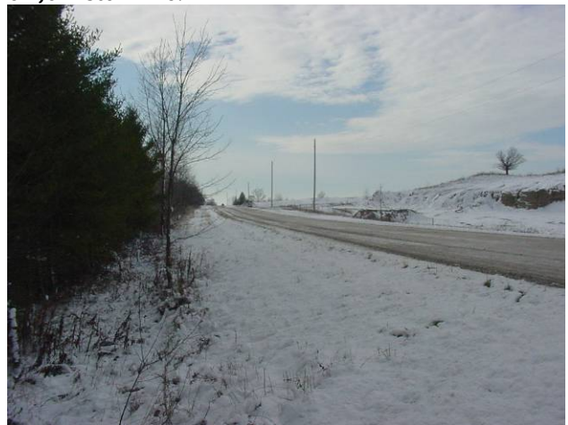
Plate 90: view to southwest, fill slope disturbance along Johnston Line.
