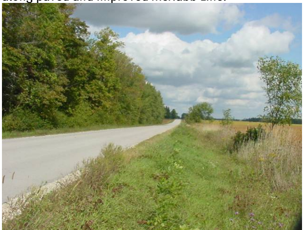
Plate 47: view to northeast, ditch and fill slope disturbance along paved and improved McNabb Line.
