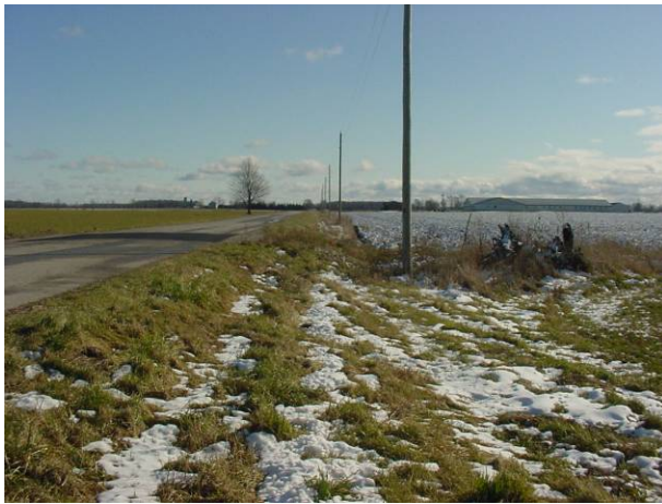
Plate 7: view southeast, fill slope disturbance along paved and improved Bridge Road.
