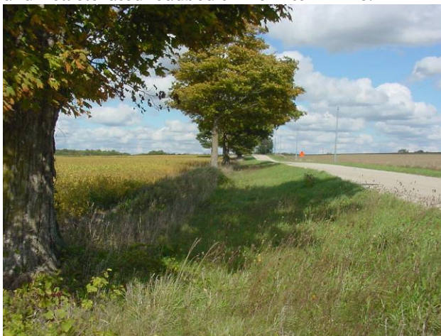
Plate 87: view to northeast, fill slope and ditch disturbance along Johnston Line.
