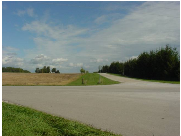
Plate 32: view to northeast, visible fill slope disturbance, adjacent to northwest side of Manley Line.
