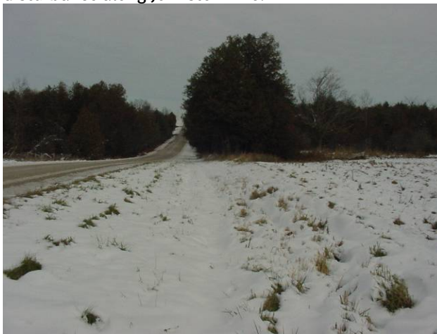
Plate 89: view to northeast, ditch and fill slope disturbance along Johnston Line.
