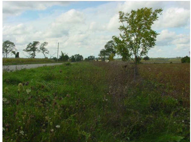
Plate 86: view to northeast, fill slope along gravelled and well elevated roadbed of Browntown Line.
