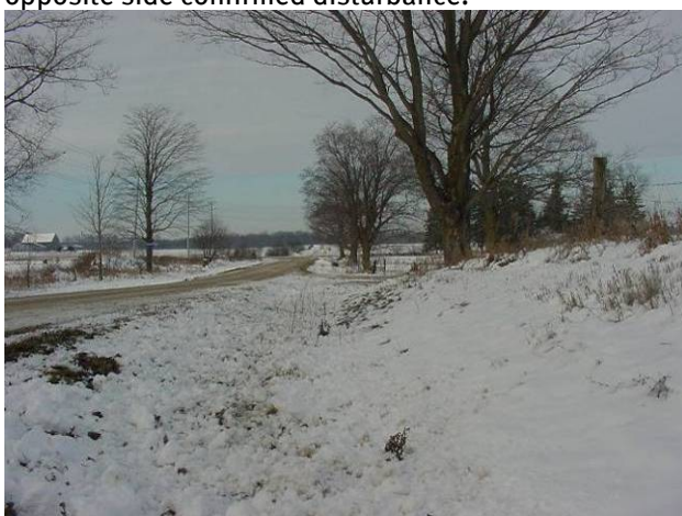
Plate 107: view to northeast, road cut, slope & ditch disturbance along Centre Line Road south of intersection with McDonald Line, near farmsteads.
