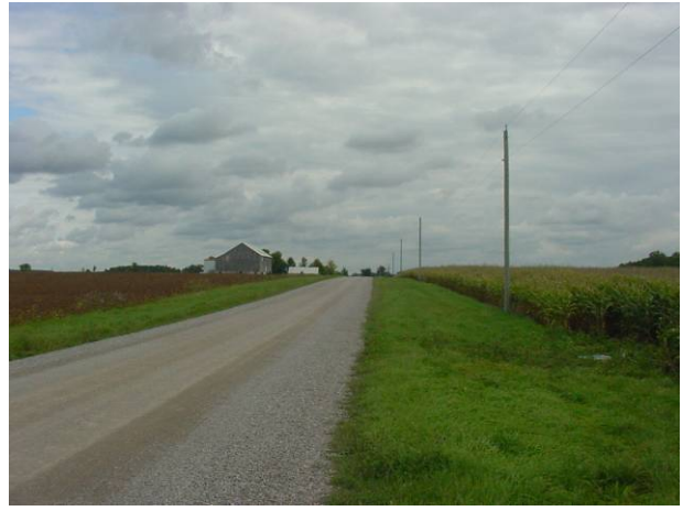
Plate 16: view to northeast, wide, gentle fill slope disturbance on southeast side of Manley Line.
