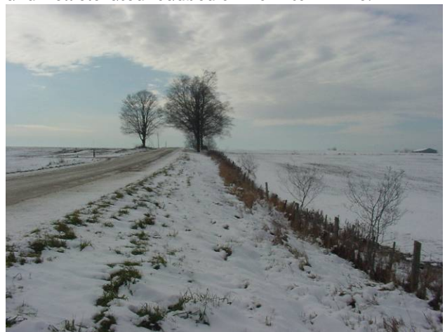
Plate 88: view to southwest, fill slope disturbance on Johnston Line.
