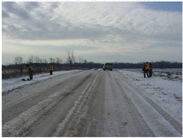
Plate 82: view to southwest, 5m interval test pits on southeast side of McNabb (fill was screened). Ditch on west.
