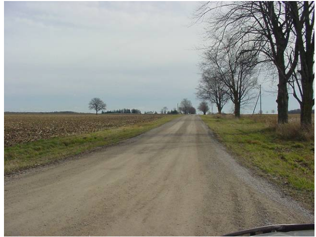
Plate 38: view to southeast, fill slope and shallow ditch disturbance along Canada Company Road.
