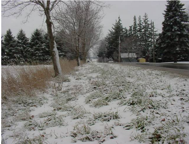
Plate 55: view to southwest, fill slope disturbance along southeast side of McNabb.
