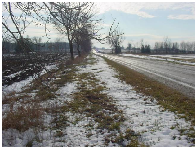
Plate 66: view to southwest, fill slope disturbance. Abandoned rail bed at tree line in distance.
