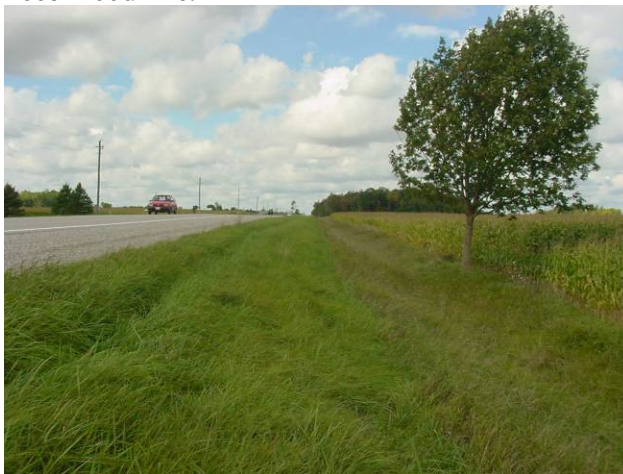
Plate 41: View northwest, fill slope and ditch disturbance along paved and improved Blyth Road.
