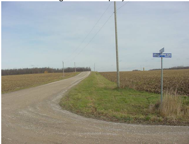
Plate 39: View northeast, fill slope disturbance along Beechwood Line.
