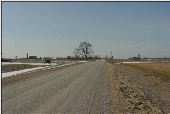
Plate 11: View to south-southwest along Beechwood Line at intersection with Summerhill Road. Shallow ditches, elevated roadbed, and level terrain.
