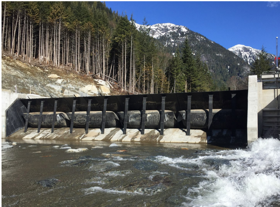
The fully inflated weir at the Chickwat intake in March 2018.
