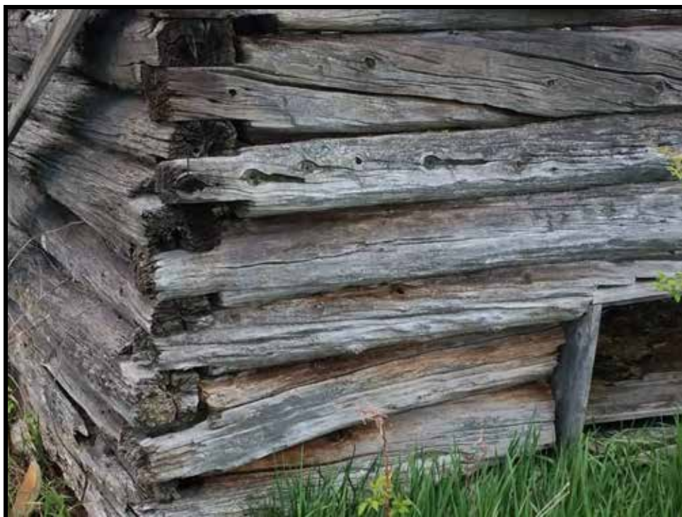
Image 41: Detail of Dovetail Corner Construction (Photo taken on May 19, 2016; Facing North)
