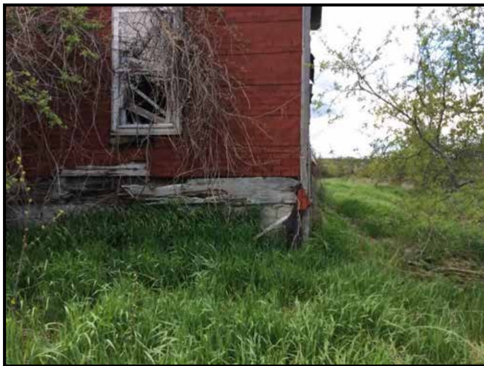
Image 14: Detail of Clapboard under Insulbrick of 697 Hinch Road (NAP021) (Photo taken on May 19, 2016; Facing North)
