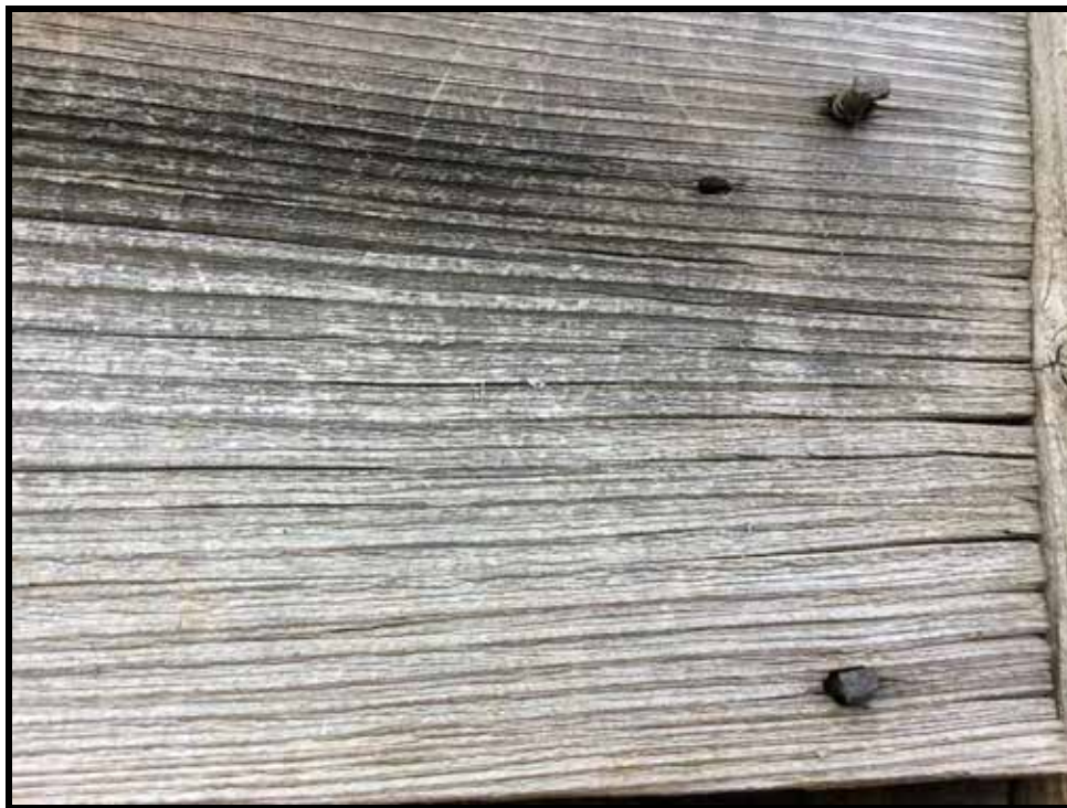
Image 20: Detail of Square Cut Nails used to Build 697 Hinch Road (NAP021) (Photo taken on May 19, 2016)
