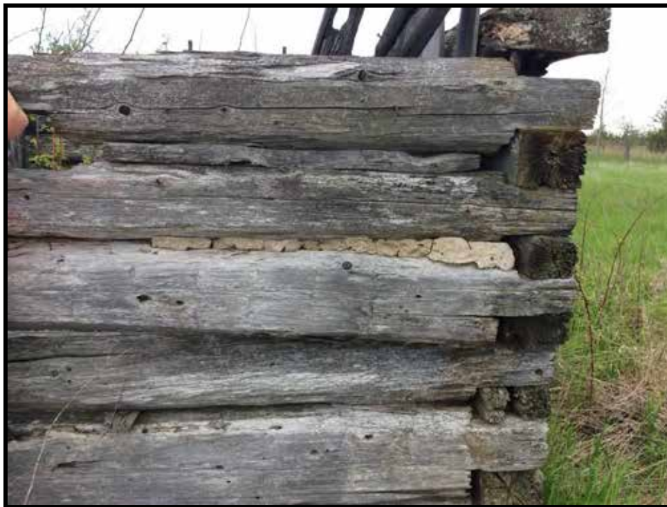
Image 40: Detail of Chinking between Hewn Logs (Photo taken on May 19, 2016)
