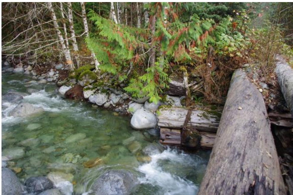
Figure 9. Looking at RL upstream bridge abutment. Channel is beginning to form a pool and outflank abutment, indicating a more sinuous form may be imposing on the previously straightened channel.
