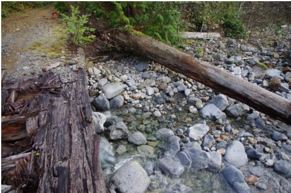
Figure 7. Evidence of bridge damage on RL downstream abutment caused by recent high flow events. Bridge opening is likely undersized for extreme flows.
