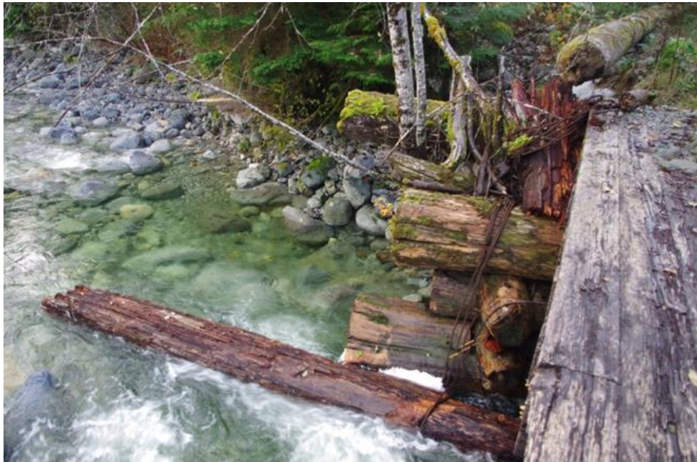
Figure 8. Downstream RR bridge abutment where channel is scouring around abutment possibly due to large boulders and a log on RL forcing flows to RR. Deepest pools in the reach are formed by scour at base of bridge abutments.
